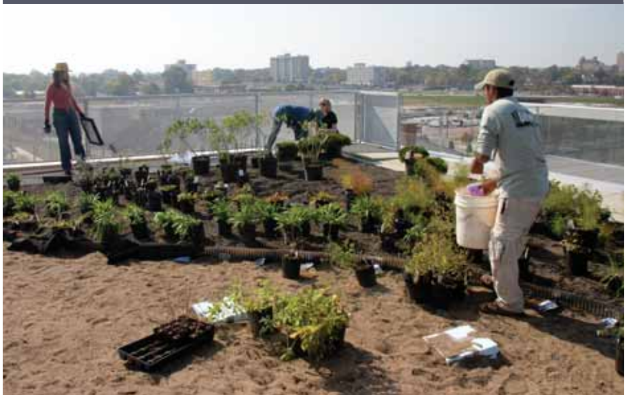
GroWild's new green roof mix is 75 percent mineral-based and 25 percent organic matter.
