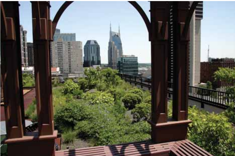
The Nashville condominium green roof after completion
