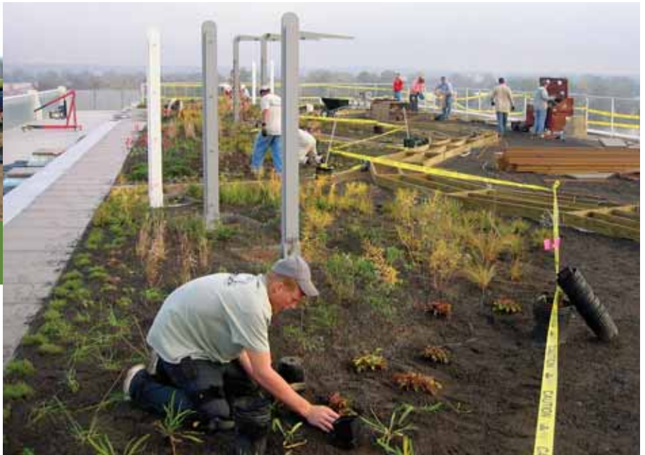
The green roof on the Clinton Presidential Library begins to take shape.
